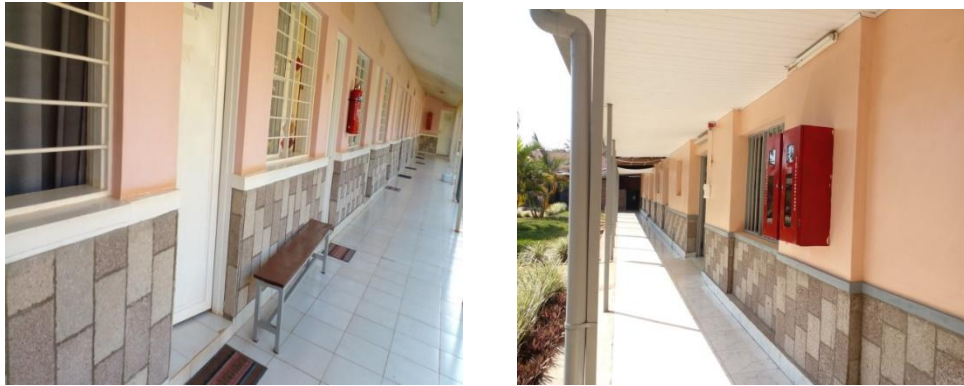
#~~~Outside walls after maintenance and dampness correction with Duhange wall tiles~~~#
