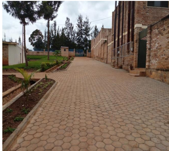
#~ Road after construction~#
