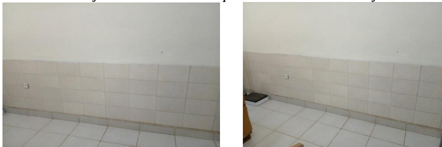
#~~~Inside walls after maintenance and dampness correction with ceramic floor tiles~~~#
