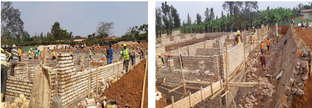
Figure 18: Construction of the first partition of Ndera rehabilitation home care
