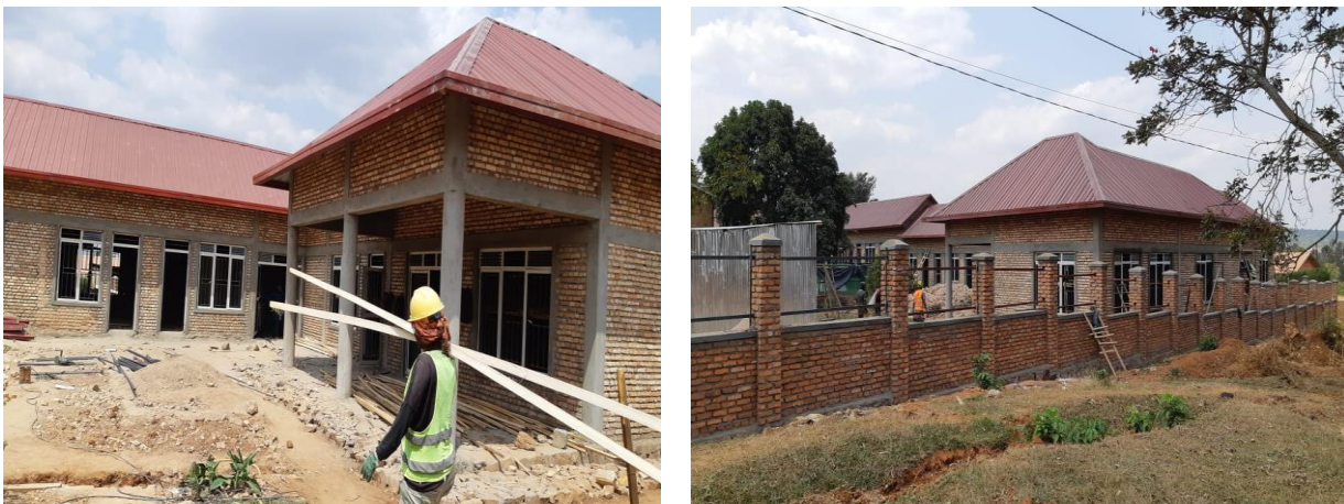
Figure 17: Construction of Residential home for hospital partners at CARAES Ndera
