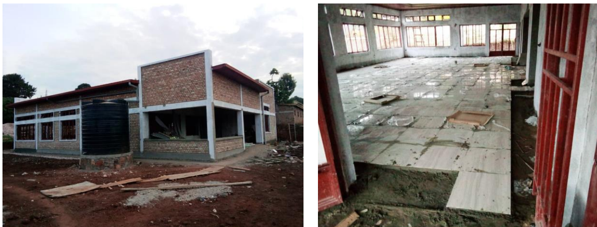
Figure 19: Construction of Occupational Therapy service at Caraes Butare
